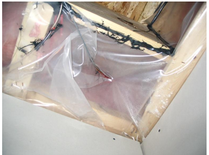
Install security wiring before insulating.
